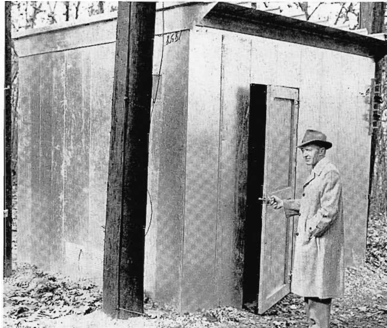
FIG. 14. Pat Flanagan, Administrative Director of Radio and TV, at door of typical Armco sheet steel pre-fab building used at relay sites.
