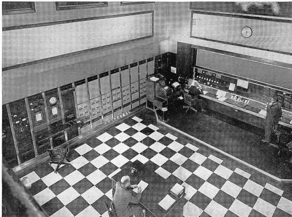
FIG. 3 (top). This picture (reproduced from an illustration in BROADCAST NEWS No. 3, April 1932) shows how the old Radio-Master Control of the Chicago NBC Studios looked in the days when it was the awe-inspiring wonder of the just-dawning electronic age. Nostalgic old-timers will recognize (but not weep for) the rows and rows of battery-operated "speech input" equipment. Battery-charging equipment alone required a control panel (balcony) larger than that of a 50 KW transmitter.
