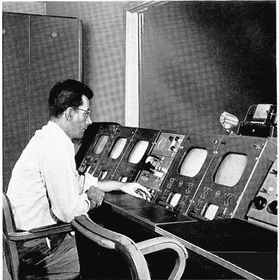
Controls for the vidicon chains are located here in the master control room. The second and third monitors from the left are the vidicon master monitors. Their housings also enclose the camera remote control panels. Both master monitors and console housings are part of the station's original iconoscope equipment.
