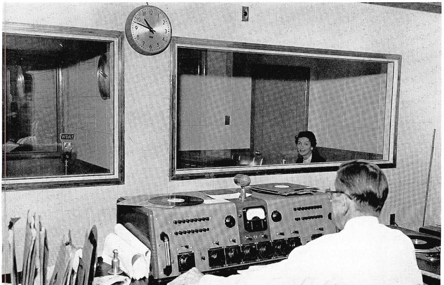
FIG. 3. View of studios and studio control. Studio "A" on left and Studio "B" on right. RCA 76B audio consolette (foreground) has given WDAS many years of dependable service.
