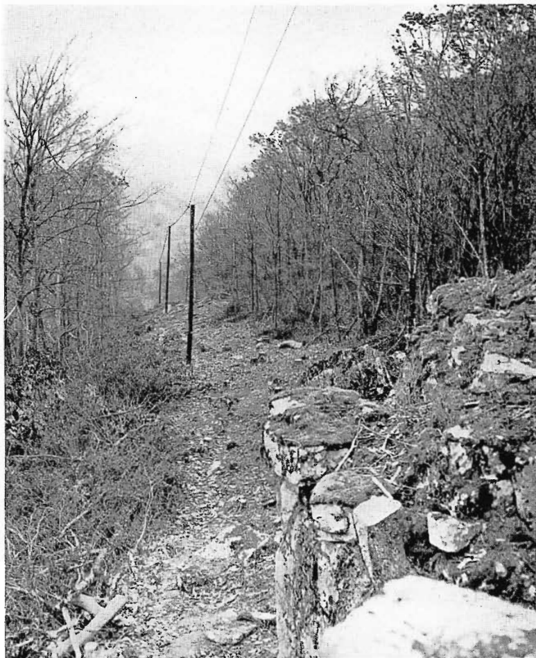
FIG. 17. Power line 1.25 miles long was built to serve installation on Dismal Peak.
