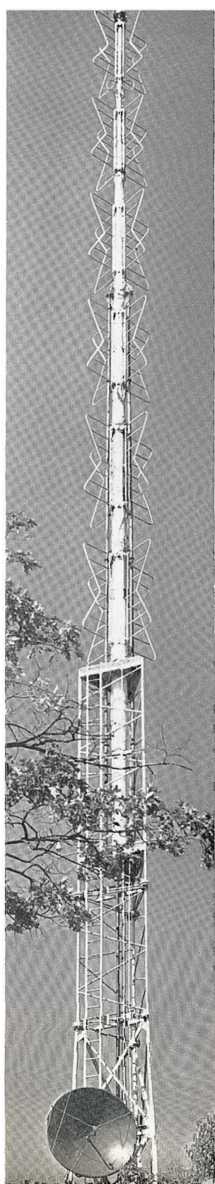
FIG. 14. Tower is 100 feet high and supports an RCA 6-bay Superturnstile 82 foot antenna.
