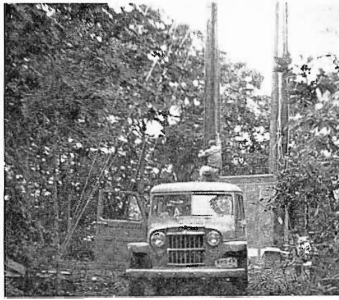
FIG. 11. Construction of relay station at Dismal Peak, Virginia.
