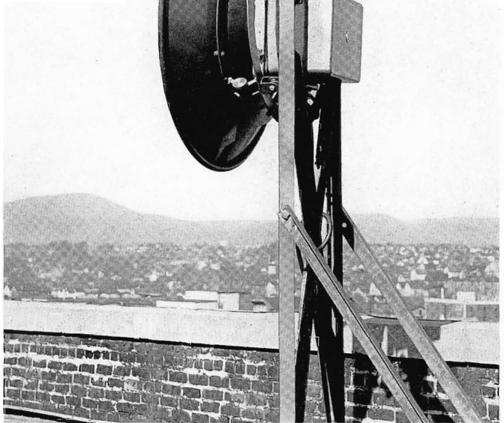
FIG. 7. Side view of microwave installation at Roanoke terminal showing 4 foot parabolic reflector with head end transmitting equipment and angle iron supporting frame.
