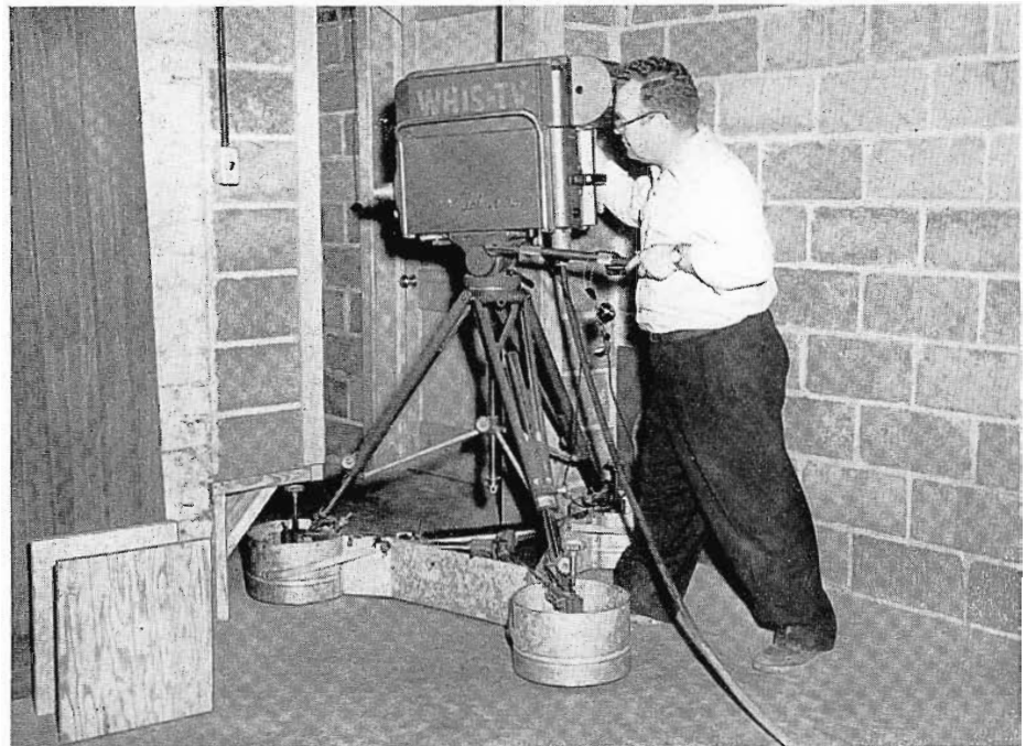
FIG. 5. Note novel construction of doorway where door jam meets floor in order to permit passage of camera dolly. Removable "boot" is shown at lower left. This is put back into position after camera has passed through.
